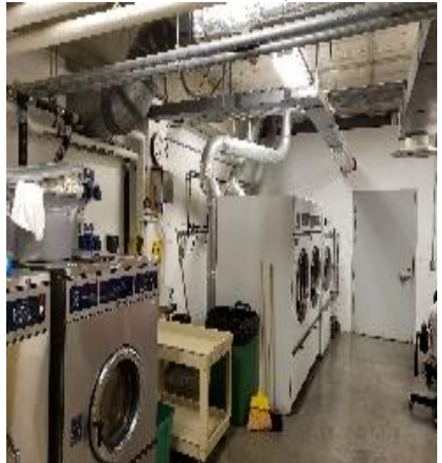
Exhibit V.5. Drafts and Dryer Vents
